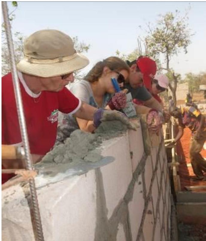
We just about finished the sand barrowing today, and the block laying for the walls reached shoulder height on all but the front (and most
